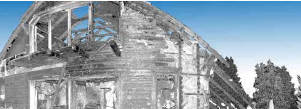
3D point cloud of a burnt restaurant
